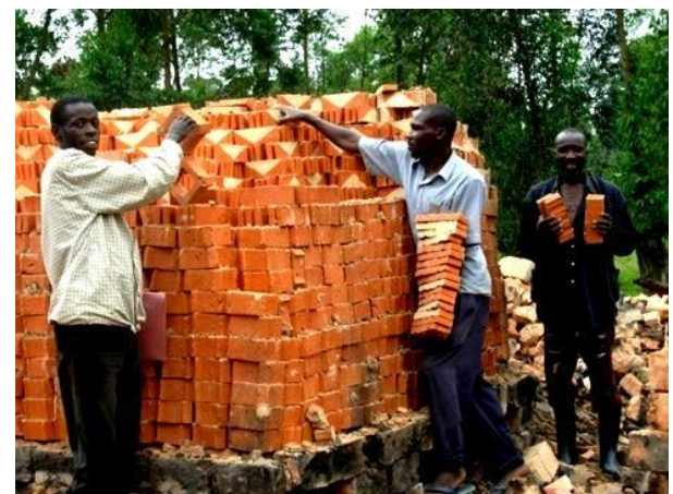
Figure 20. Offloading and selecting face bricks and decorative grills.
