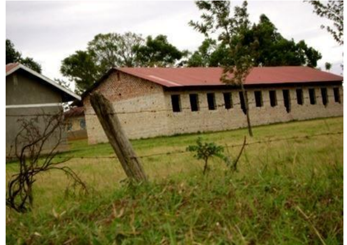
Figure 9. UPE building constructed with bricks contributed by parents.
