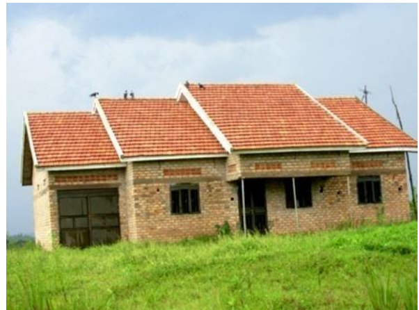
Figure 12. A house built and roofed using locally made bricks and tiles.
