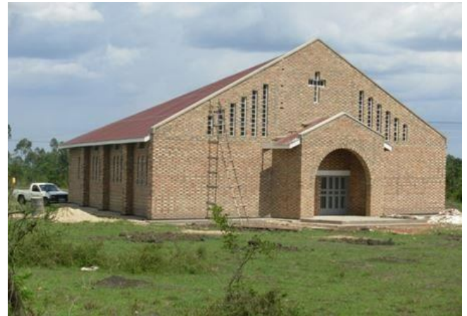
Figure 10. A church under construction using bricks.
