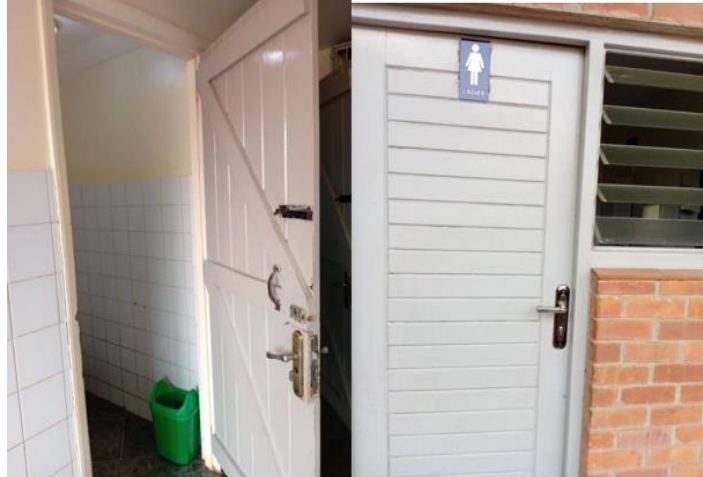
Figure 4. Labeled Toilets at Campus A
