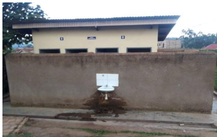
Figure 6. Non-water Borne toilet at Campus B
