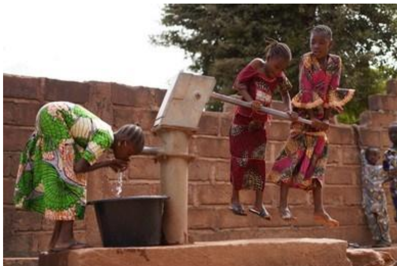
Figure 2. 12 : Borehole prone to breakdown because of rigidity of the pumping system
