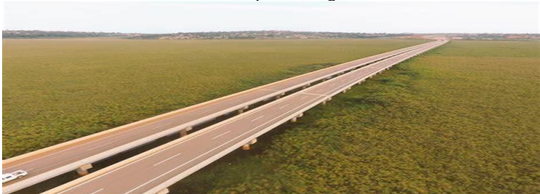
Picture 3: The Kampala, Entebbe road constructed between 2012 and 2018
