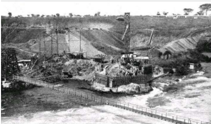
Construction of Owen Falls Dam in Jinja
