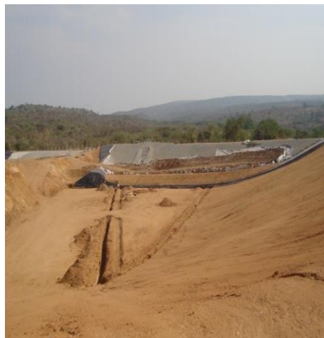
Left - Waste treatment facilities at the Enviroserve waste management Facility in Nyamasoga in Buseruka Sub-county, Hoima District. Right - A solid waste engineered land fill at the facility.
