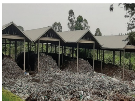
(a): Compost raw materials in windrow bays
