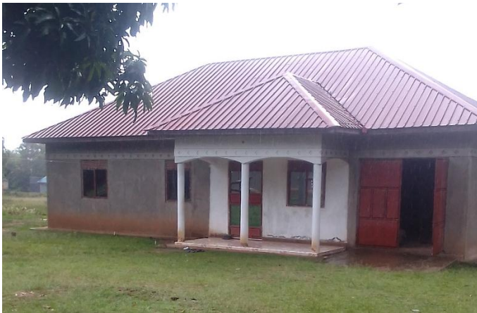
Figure 4 1: Newly Constructed Guest House at Alioce Church of Uganda, Arua Archdeaconry
