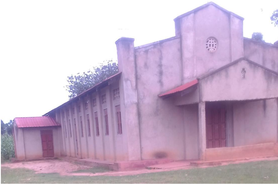
Figure 3 3: Picture Showing the New Church Structure of Oreku Church of Uganda, Arua Archdeaconry
