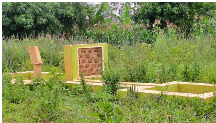
Figure 4.2 Abandoned, non- functional borehole
