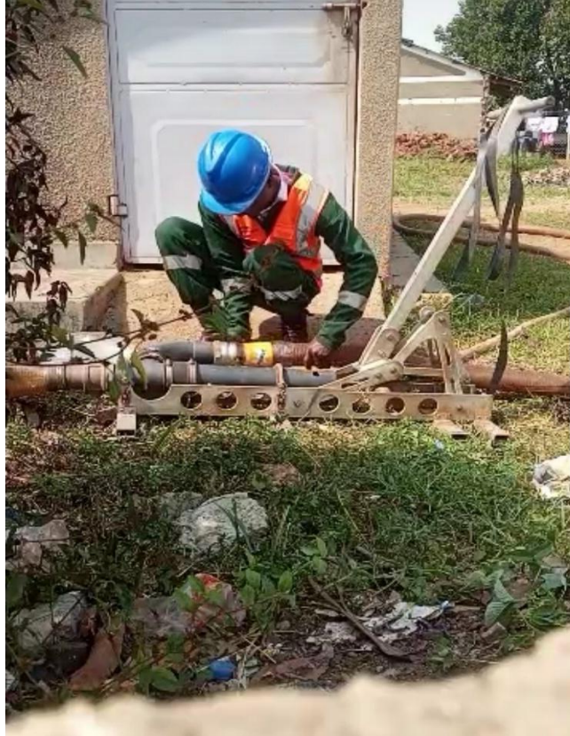
Figure 12 Hose pipes being coupled to improve on access to the containment.
