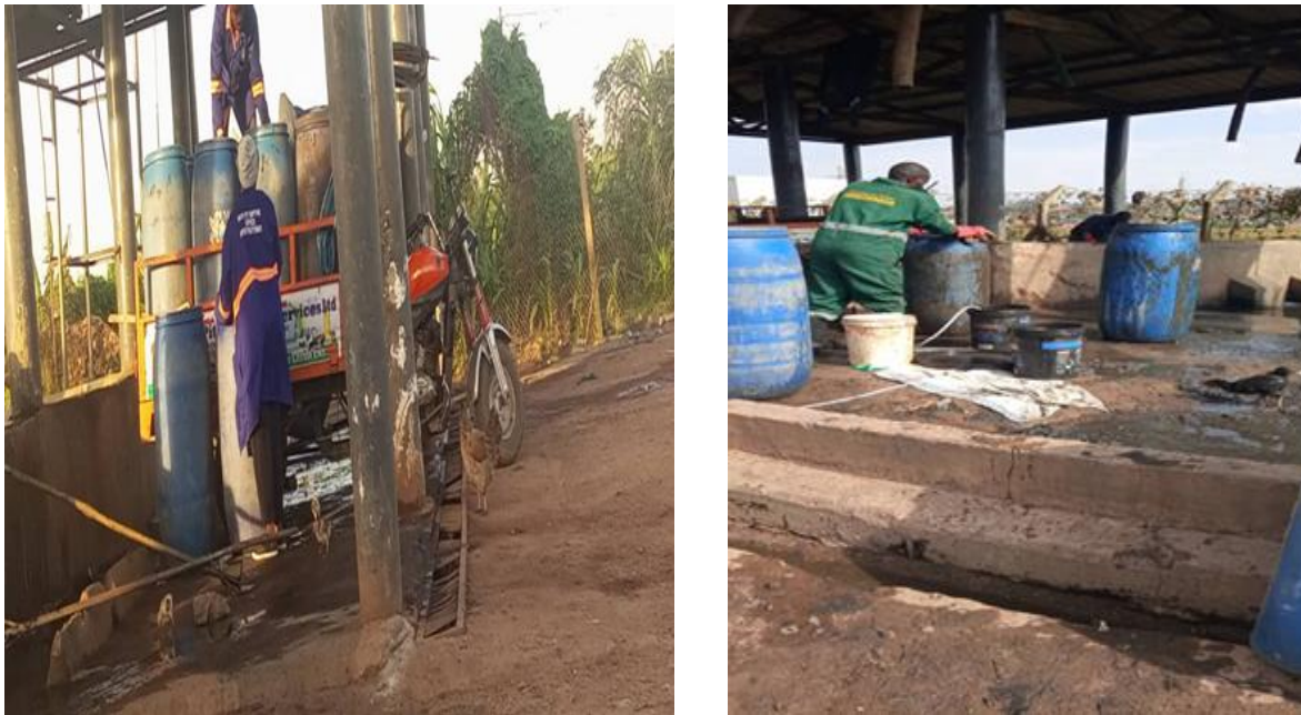
Figure 27 Offloading and cleaning drums at the FS treatment plant in Lubigi-Kampala
