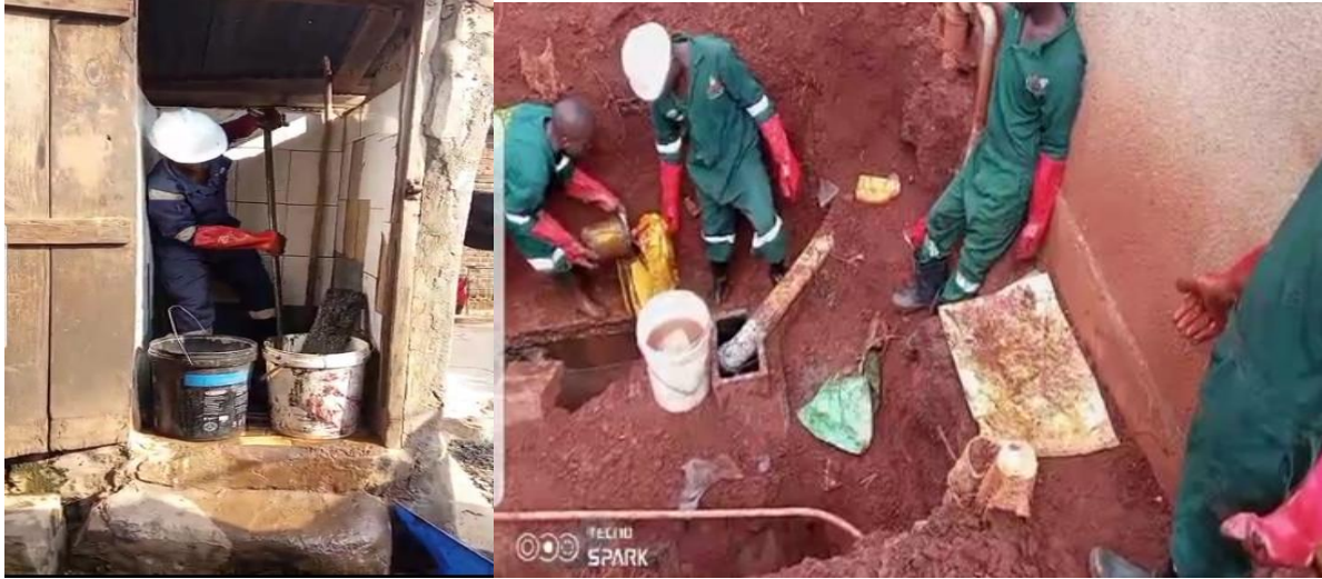
Figure 11 Gulper operator inside the containment and usage of buckets to aid the emptying process.
