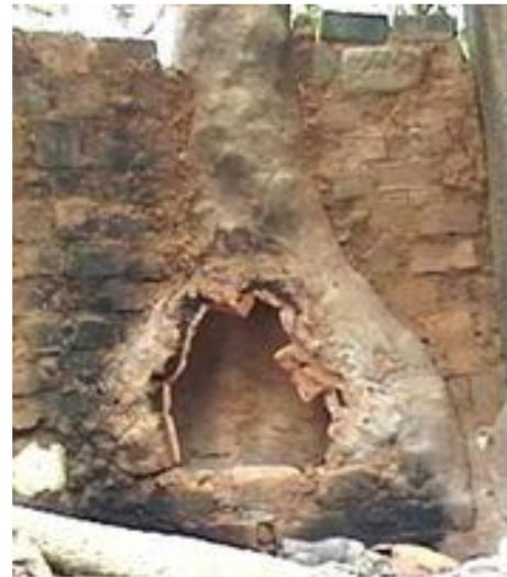
Figure 15. Locally constructed bottle updraft kiln.
